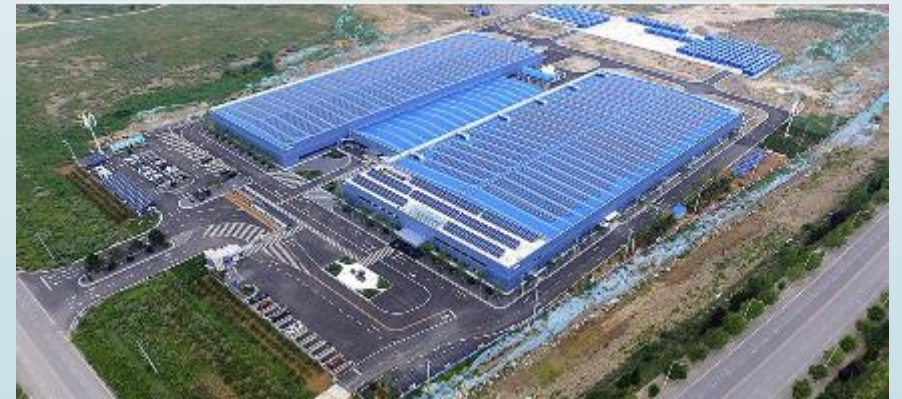
China, 200 MW flow batteries , 2017
